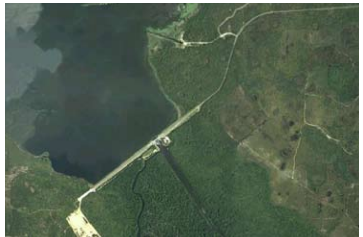
Rodman Dam on the Ocklawaha River, Google Earth
